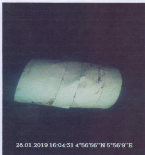
Fig D: picture taken after wrapped.
