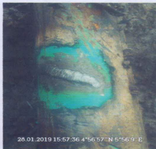
Fig B: picture taken after Patching.
